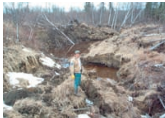
Effect of thawing of ice-rich permafrost in Alaska. Photo: V. Romanovsky
