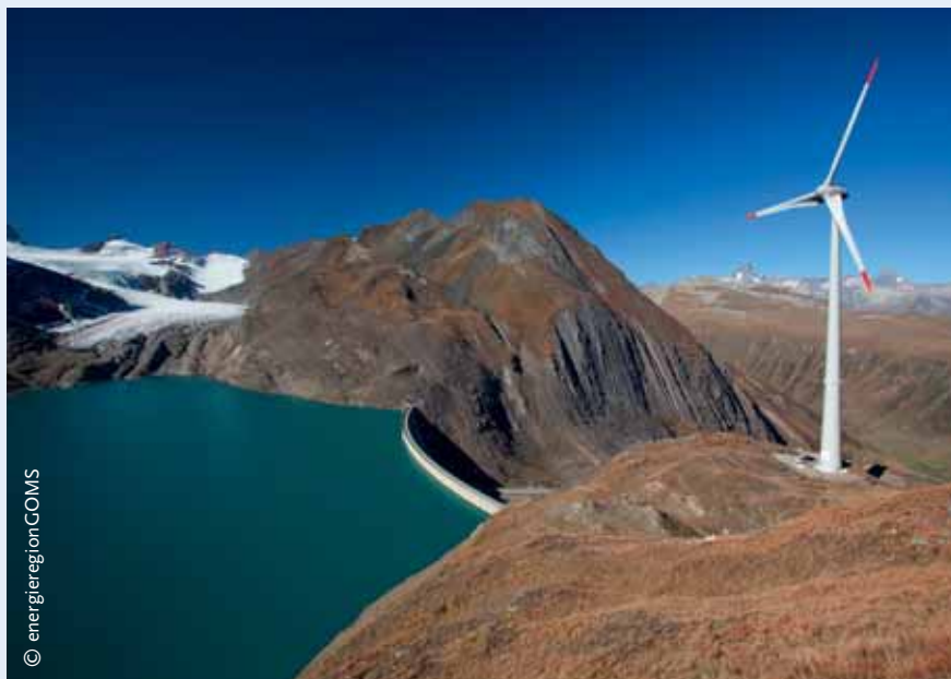
FIGURE: The highest wind generator in Europe is located at 2465 metres a.s.l. near Griespass in Switzerland. Energy research provides technological solutions for the energy transition – but it also needs to consider societal issues, such as acceptance of renewable energy production.
